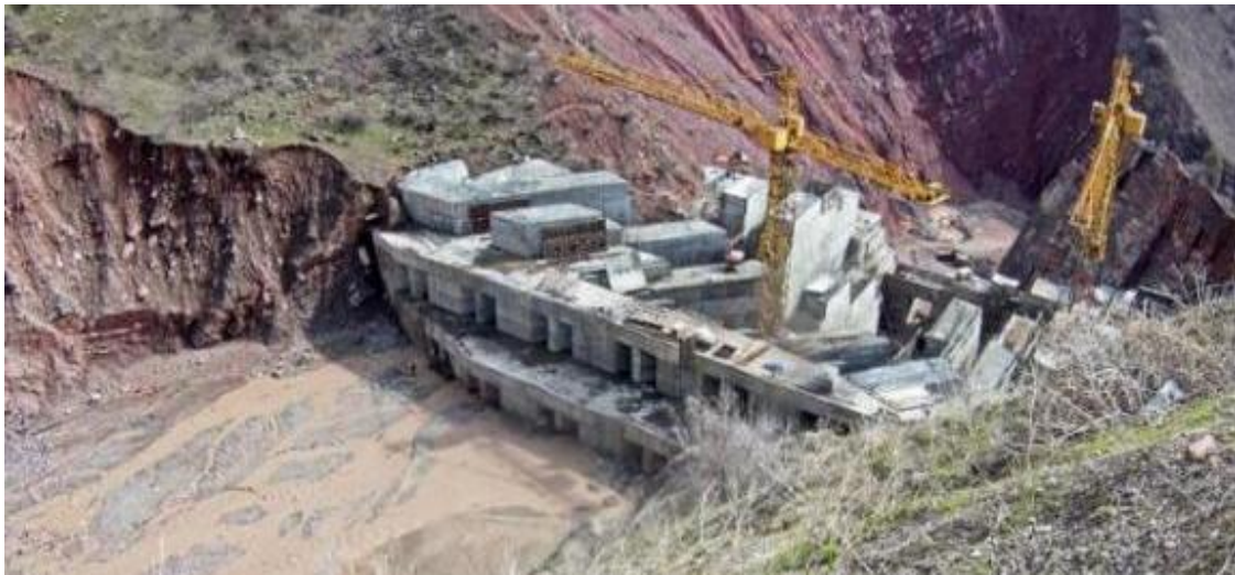
Figure 3. Construction of Existing Check Dam (2010-2015)
