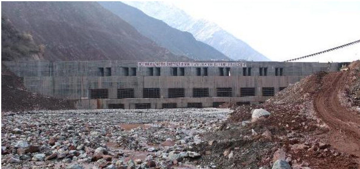
Figure 4. Upstream Face of Existing Check Dam (2026)
