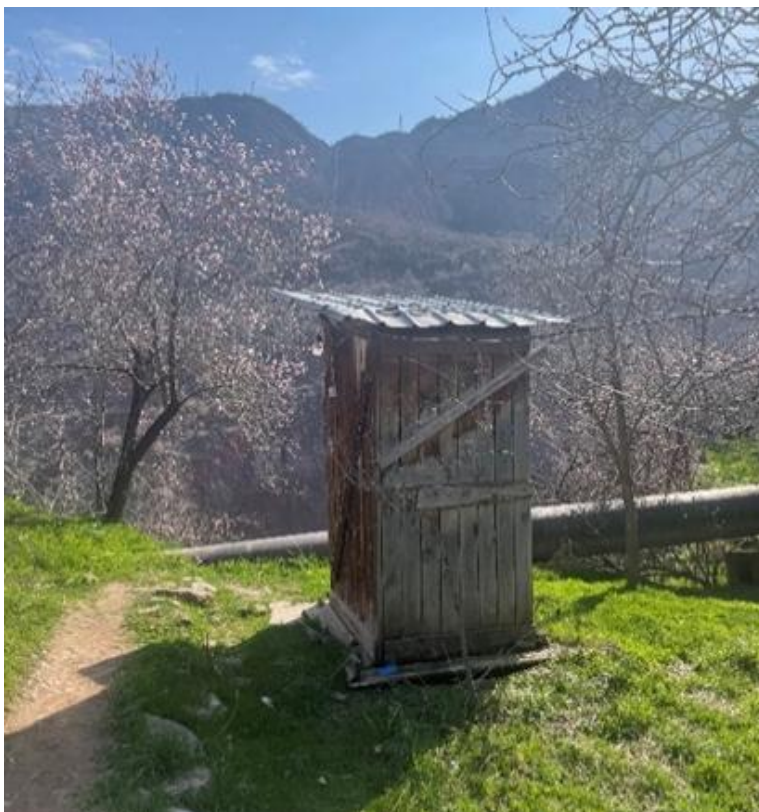
Figure 17-3 - Women's Toilets at a Workers' Camp Site within the Construction Zone (August 2023)
