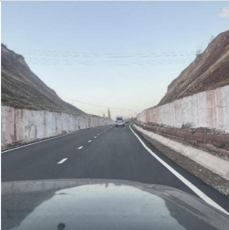
Photo 1: A well-maintained asphalt section with clear lane markings and protective barriers.
