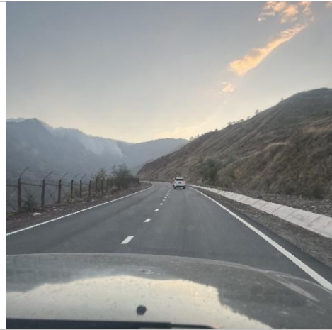
Photo 6: A well-maintained section of the Dushanbe–Rogun route with clear markings and safety barriers showcases improved infrastructure.
